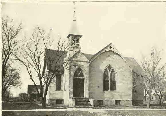
CONGREGATIONAL CHURCH, CLAY CENTER
